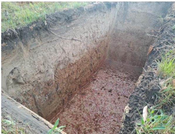
Figure 12: TP1 comprising colluvial deposits overlying pale orange residual clays, grading to extremely weathered granite as mottled clay
