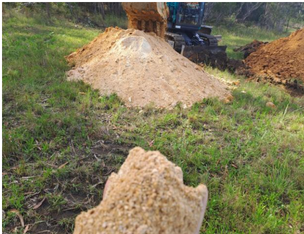
Figure 14: HW Granite excavated as gravelly sand from TP3. Excavator refusal was not encountered within limits of reach
