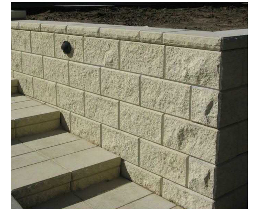
Split Face Core Filled and Reinforced Concrete Block Retaining Wall
