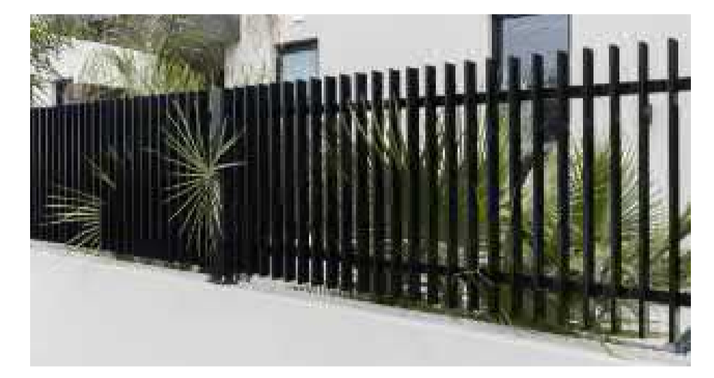
Permeable Fence Mounted to Top of Retaining Wall
