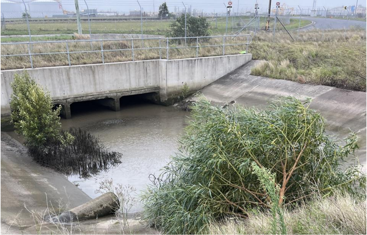
Photograph 22: Concrete drain in the north-west portion of the project site
