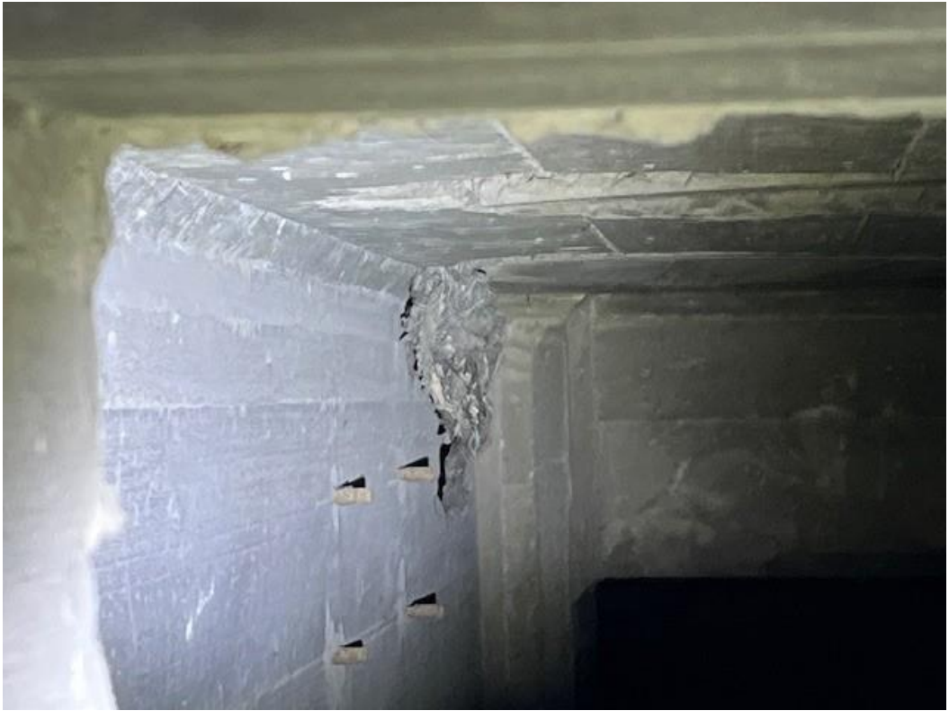
Photograph 18: The confined space via the entrances
