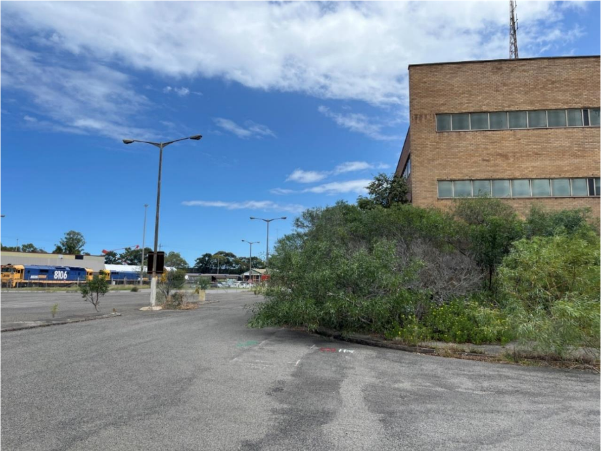
Photograph 23: Area between the Office building and the south-east drain
