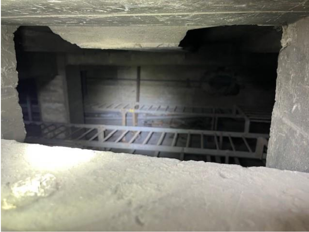
Photograph 17: The confined space via the entrances.
