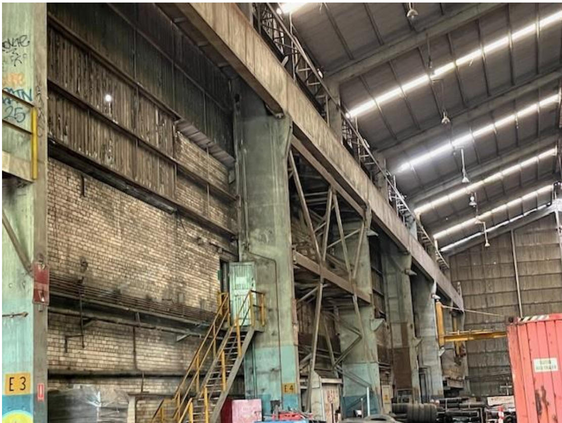
Photograph 14: Interior of Roll Shop
