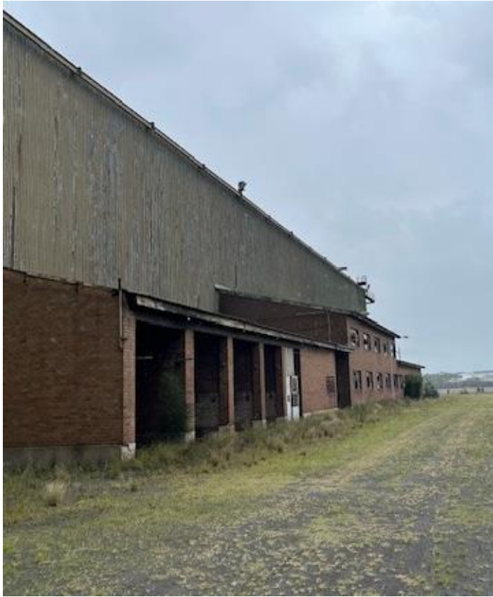
Photograph 12: Eastern exterior of the Roll Shop
