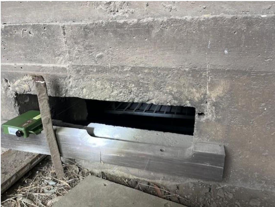
Photograph 16: Entrance to confined space indicated by yellow circle in Photograph 14.
