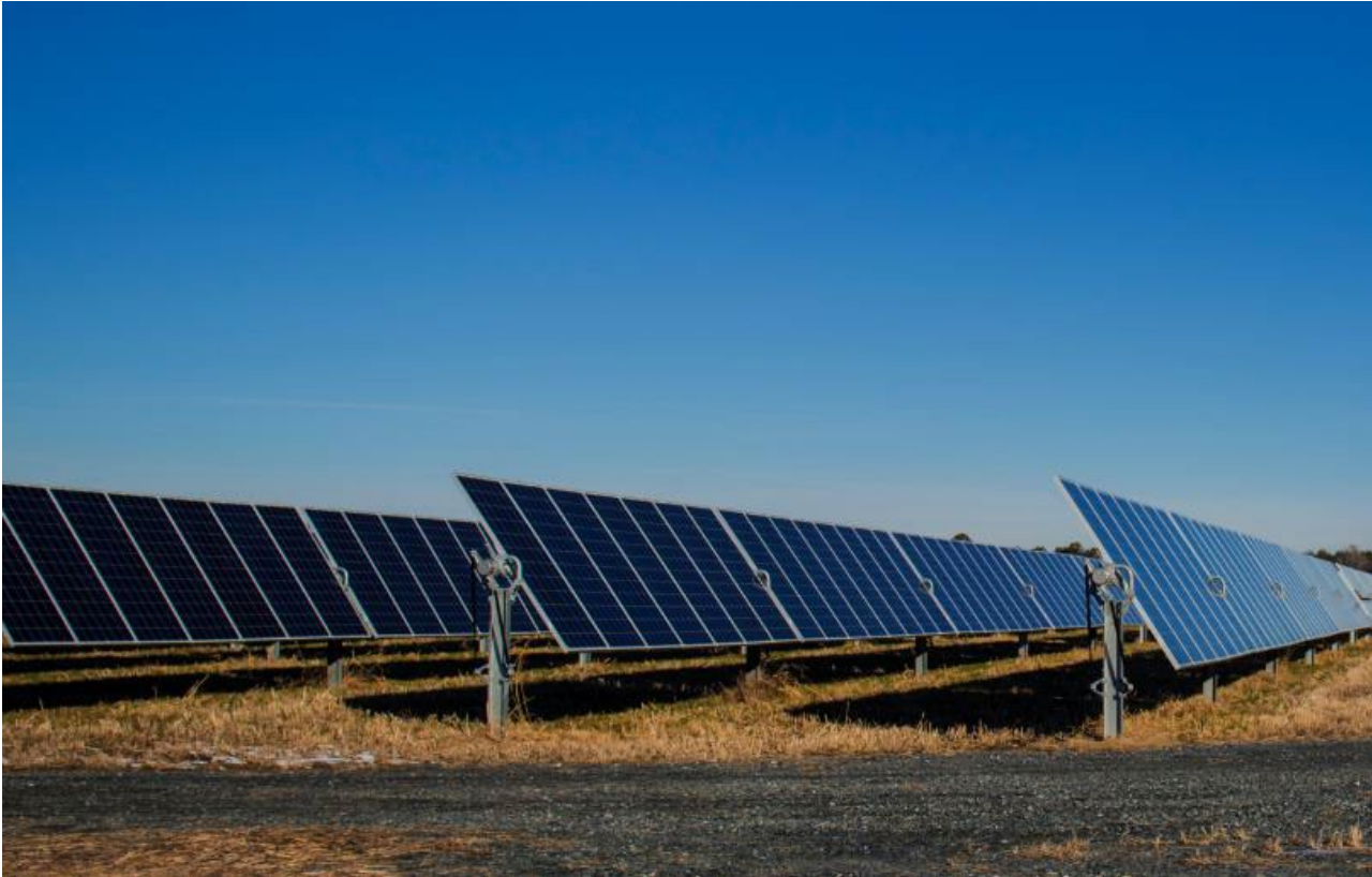
FIGURE 3-4 EXAMPLE OF SINGLE AXIS PV ARRAY
