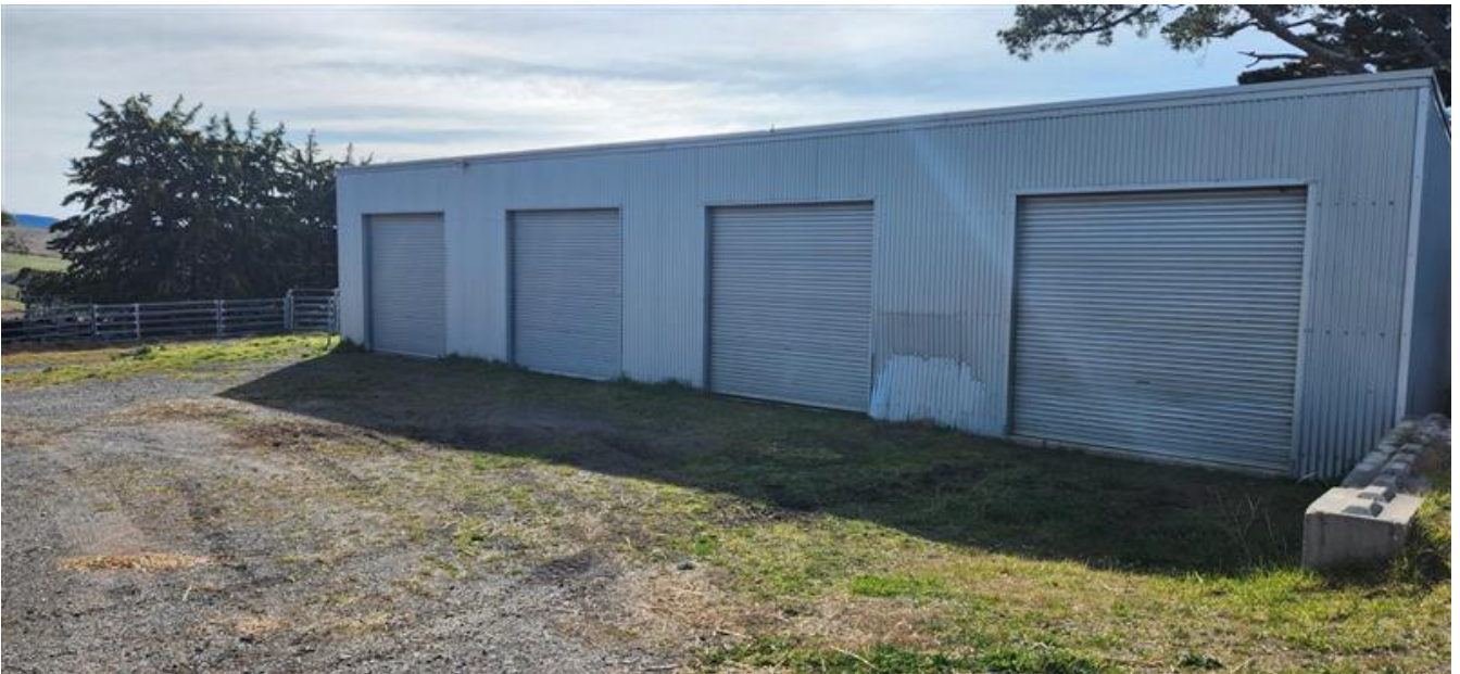
Figure 2.2 Sheds located at Cross Station
