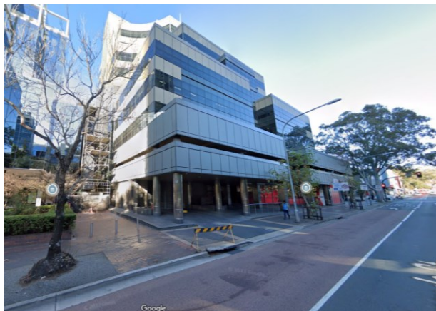
Picture 1 View of site looking west from Argyle Street.
