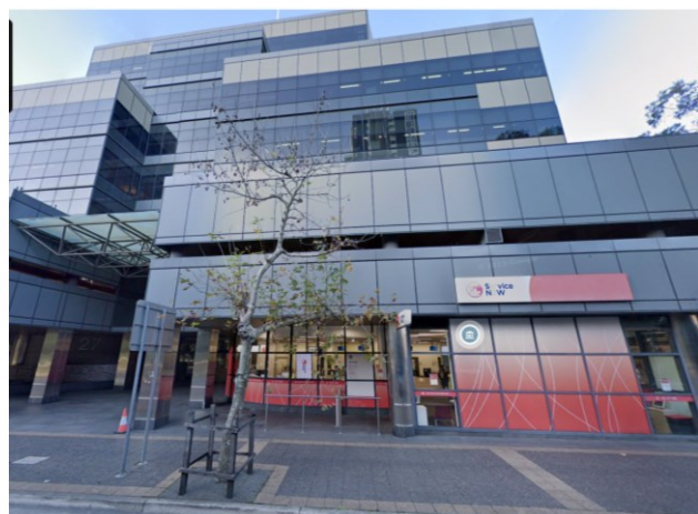
Picture 2 View of site from Argyle Street
