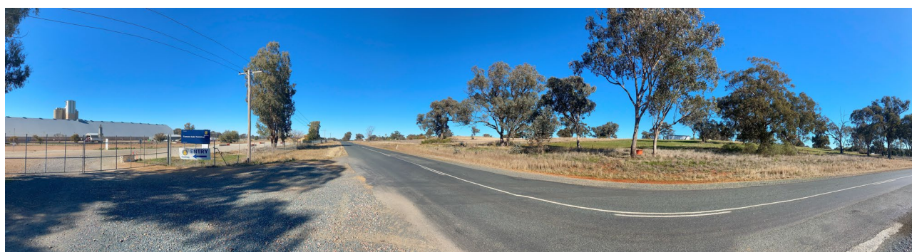
Figure 4.1 Panorama of GrainCorp Driveway Entry (left) and Project Area (right)
