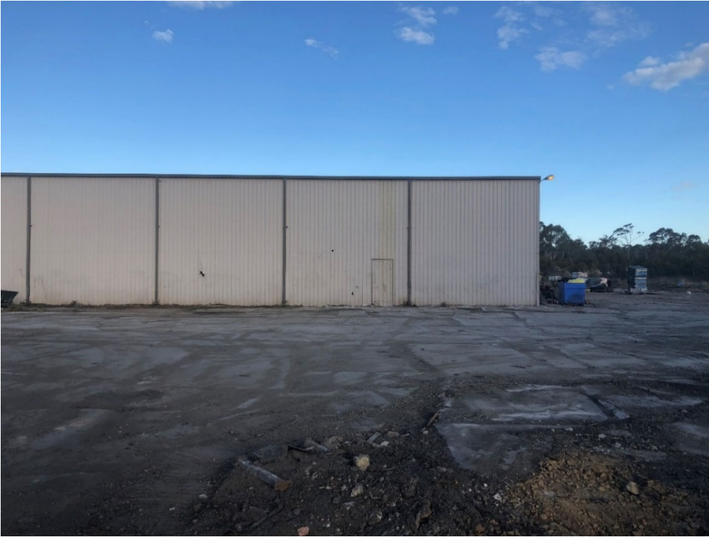
Photograph 3 Existing shed, northern portion of the site
