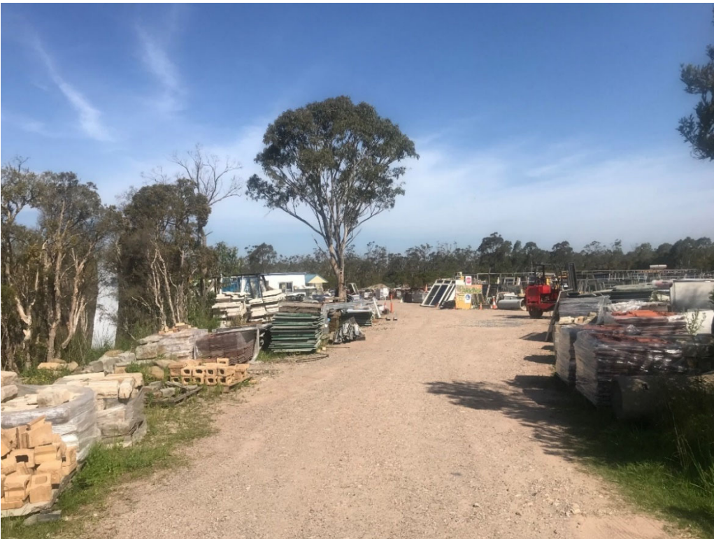
Photograph 4 Existing building materials recycling depot within the southern portion of the site— entrance off Jack Grant Avenue
