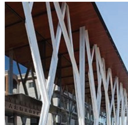
Featured 'tree' columns
