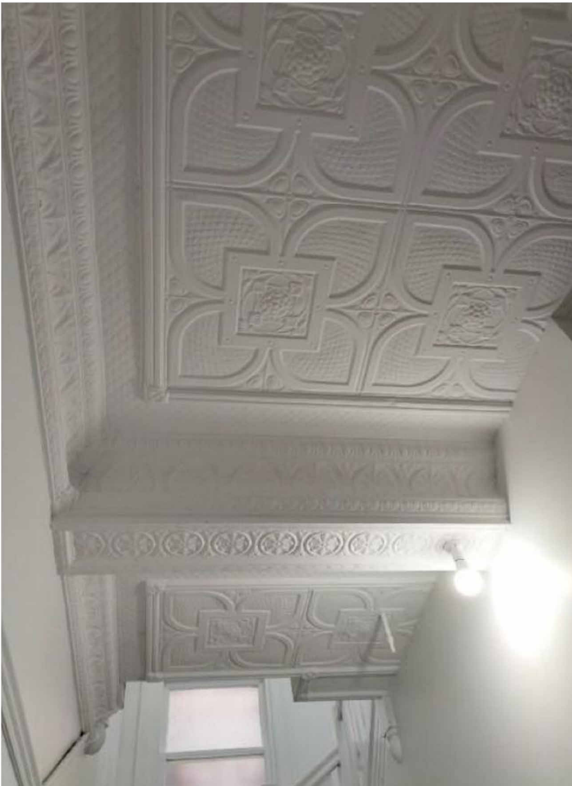
INTERNAL VIEW OF THE SIGNIFICANT PRESSED METAL CEILING IN THE ENTRANCE LOBBY
