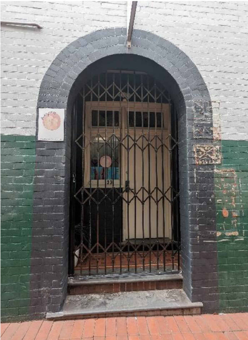
ENTRY VIEW OF THE ARCHED ENTRYWAY LOCATED ALONG THE WESTERN ELEVATION OF THE ROYAL BANK BUILDING
