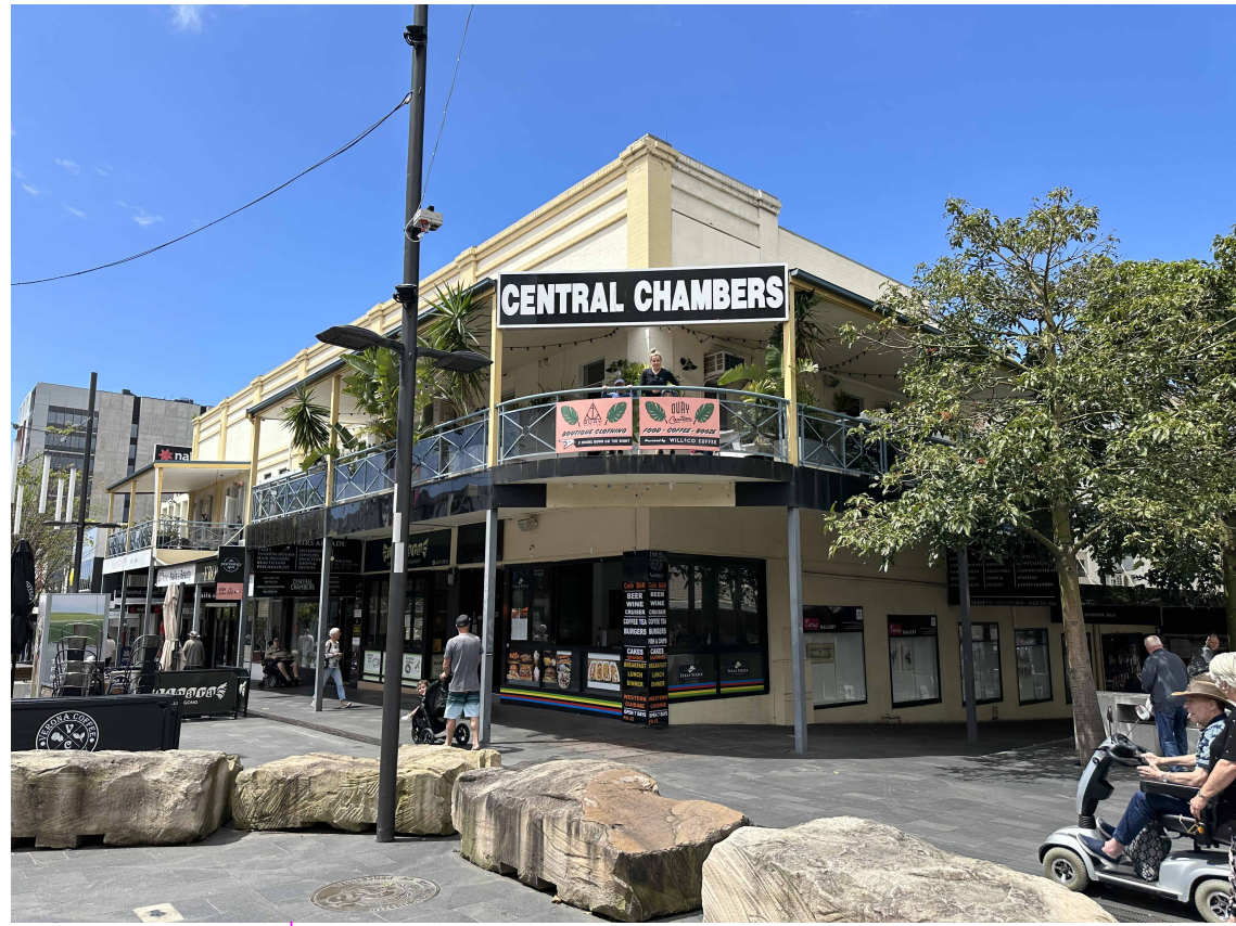
VIEW 1 - CORNER OF CHURCH AND CROWN ST LOOKING SOUTH EAST TOWARDS PROPOSAL SITE. SHOWING BUILDING CHARACTER AND CROWN ST PEDESTRIAN FOOTPATH
