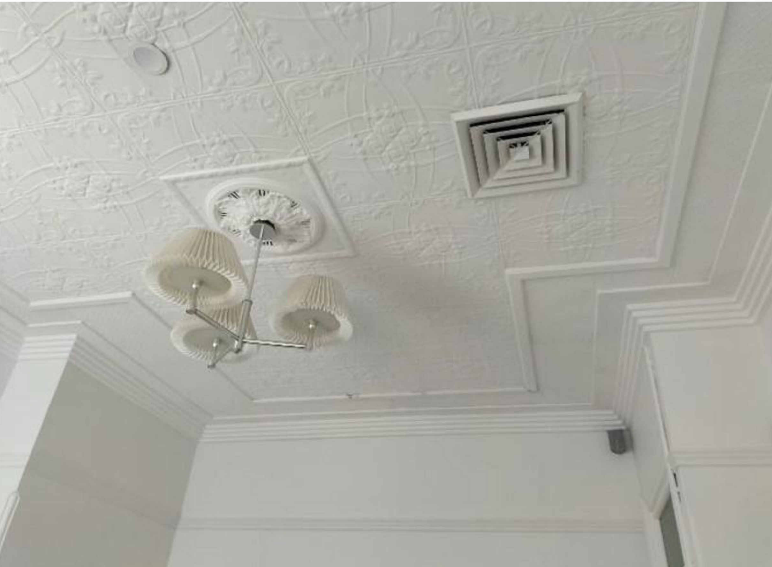
INTERNAL VIEW OF THE TENANCY ON THE FIRST FLOOR SHOWING PRESSED METAL CEILING
