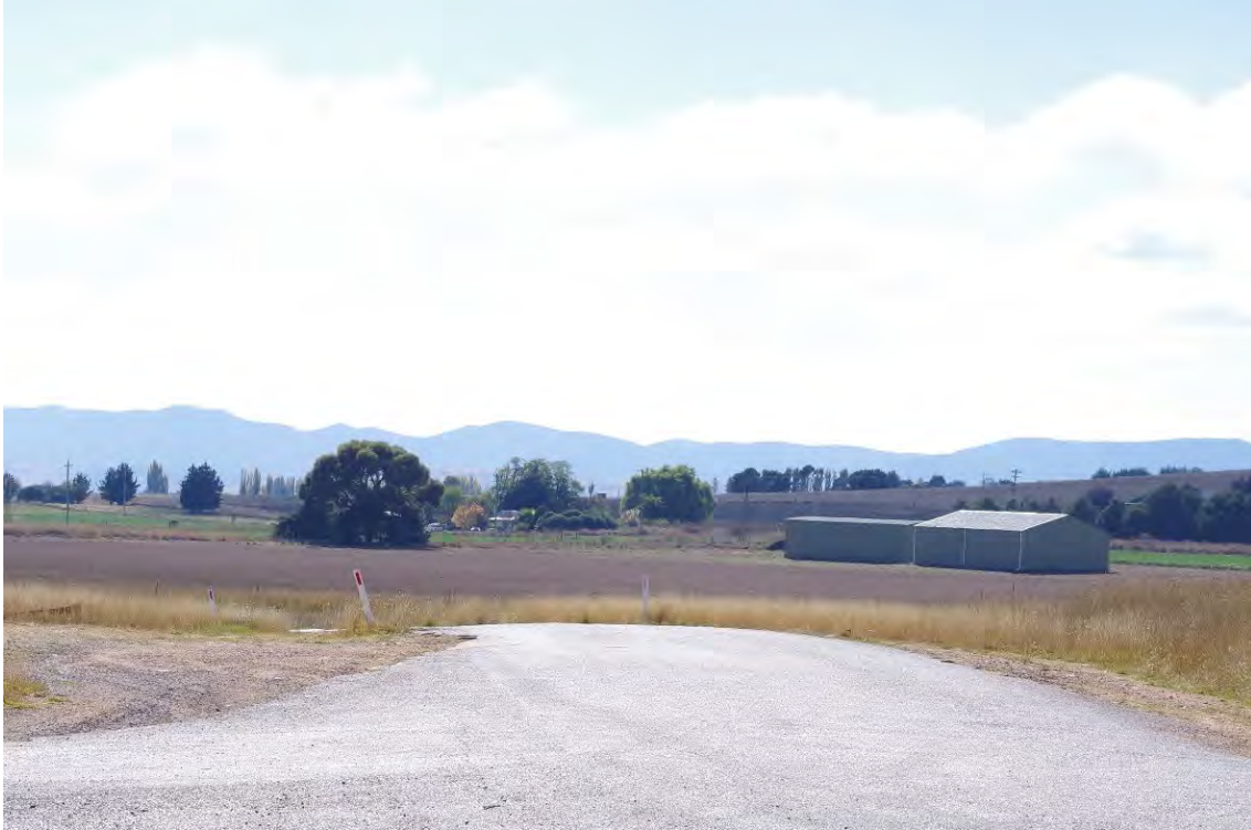
Photo 6.1 View of a sharp left turn after entering Rose Valley Road from the Monaro Highway
