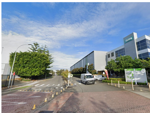
Picture 1 View of Site from outside, at Coward Street (looking south-west)
