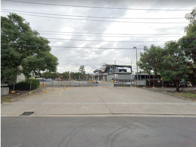
Picture 1 The site and now demolished buildings from the Crescent Street vehicular access.
