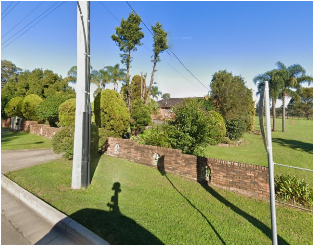
Picture 1 View of the residential dwelling at 183 Rickard Road.
