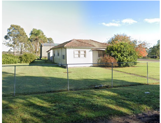
Picture 2 View of the residential dwelling at 173 Rickard Road.
