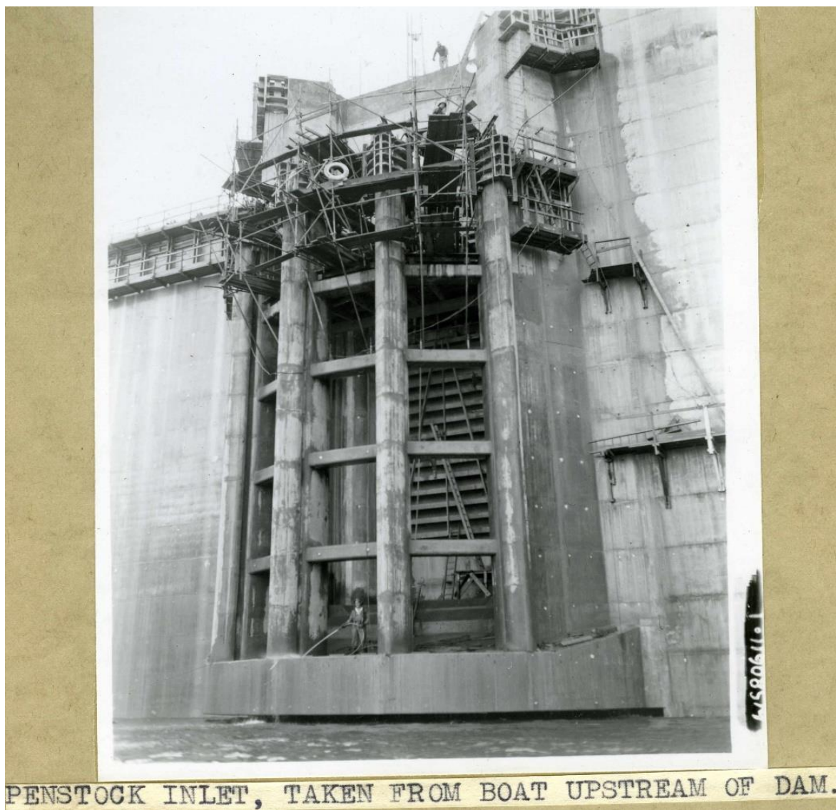
Construction photo of existing HEPS intake structure
