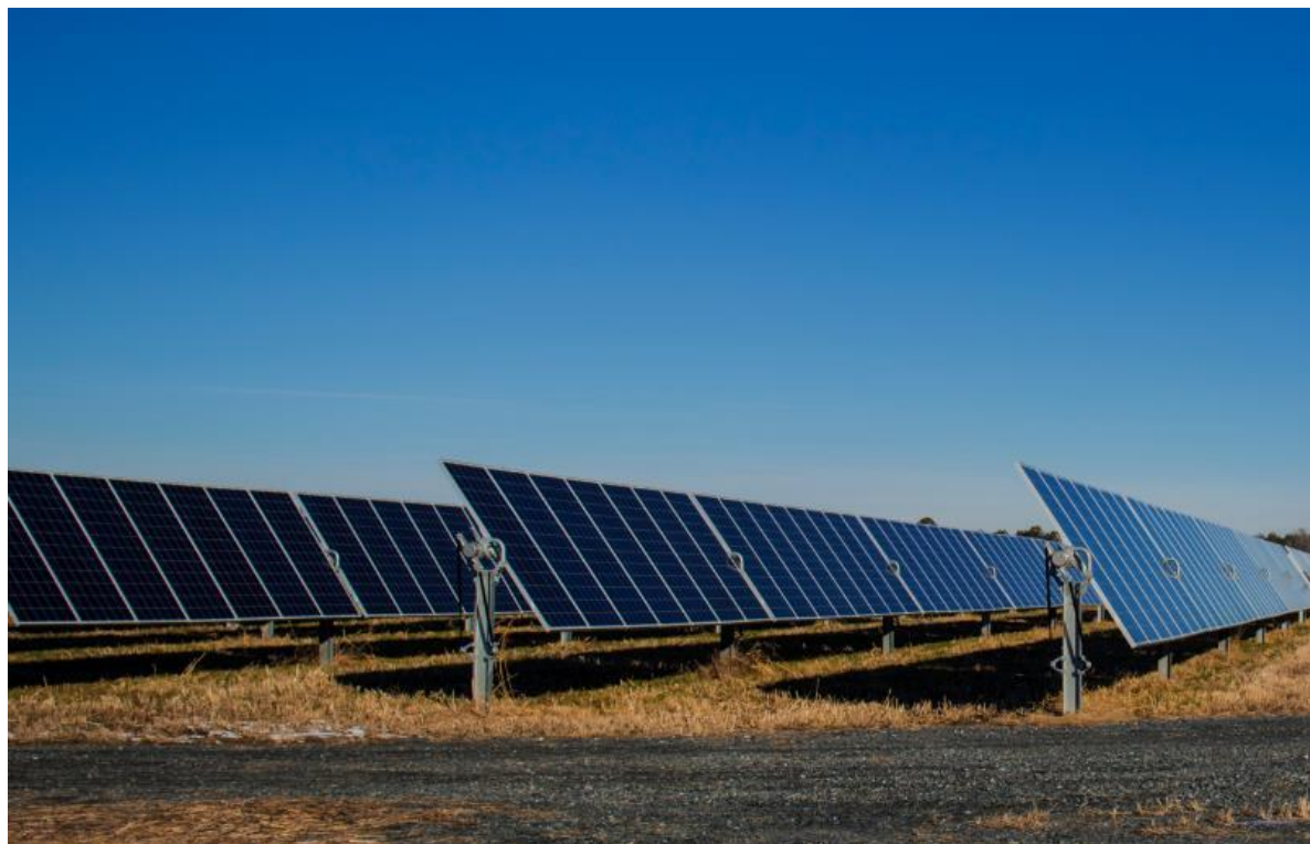
FIGURE 3-2 EXAMPLE OF SINGLE AXIS PV ARRAY
