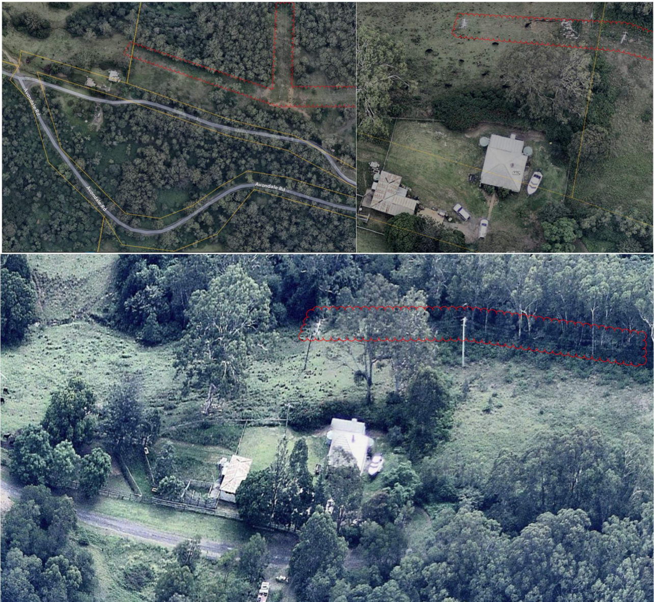
Figure 3: Existing HV overhead reticulation adjacent 662 Avondale Rd (Northern Gate location).
