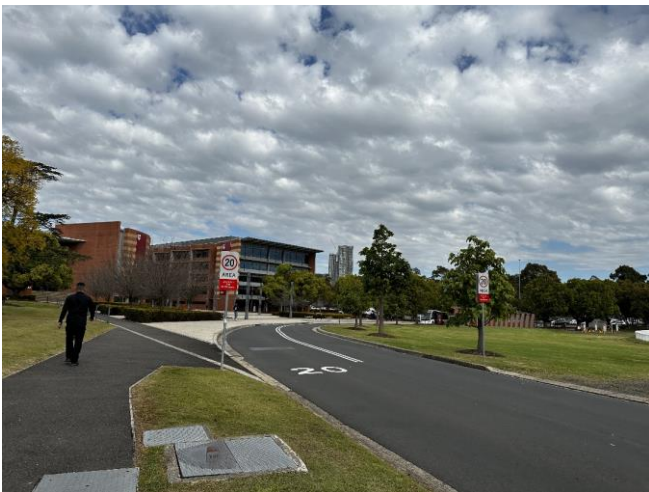
Figure 13 – View of the EB building with the existing oval adjacent
