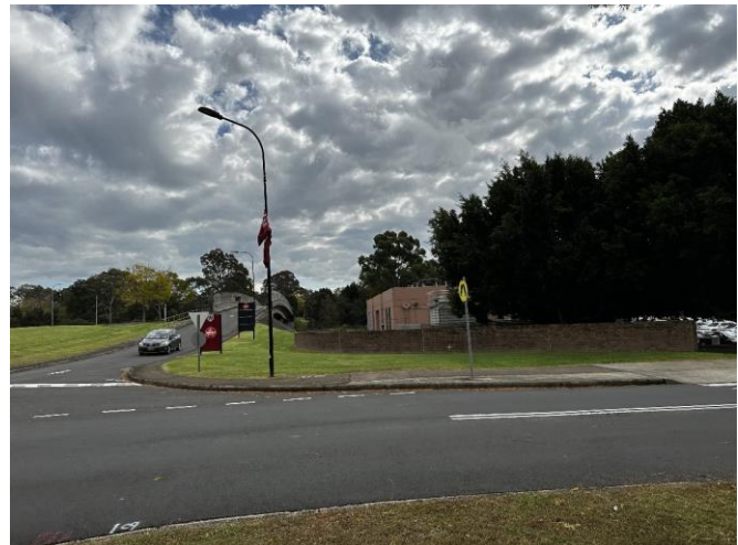
Figure 7 – Existing vehicle north-south Victoria Road overpass bridge to the west of the P1 car park site
