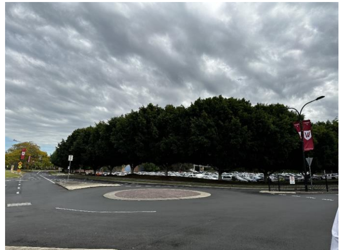
Figure 12 – Existing internal road looking north-west at the P1 Car Park
