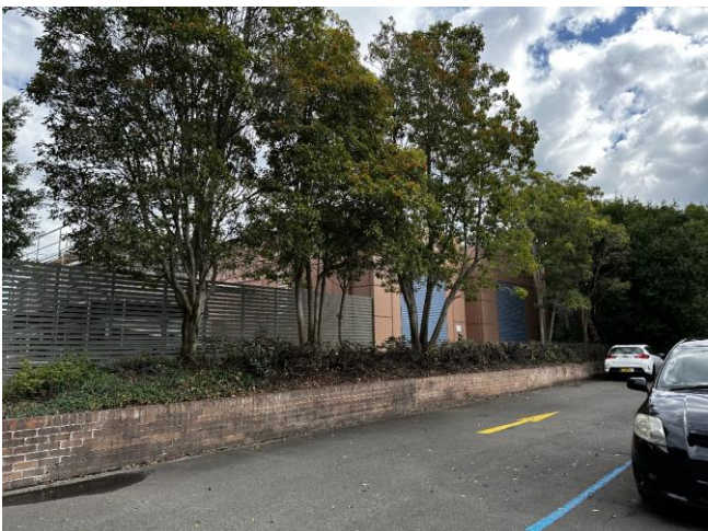
Figure 6 – Existing single storey campus central plant building contained to the west of the P1 car park site
