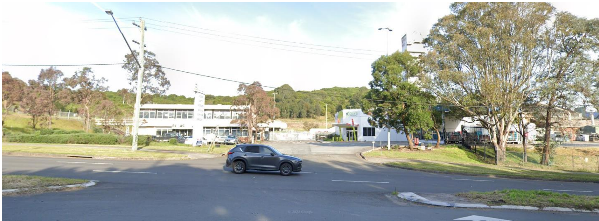
Figure 2.3 BOC site frontage and main site access
