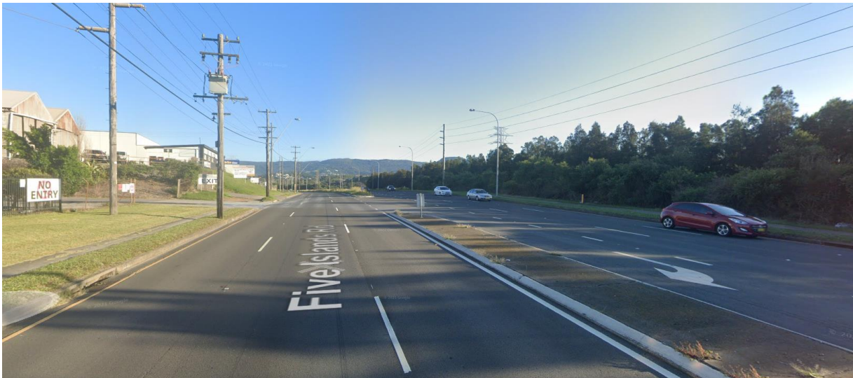
Figure 6.2 Five Islands Road, viewed northwest towards Princes Motorway Road
