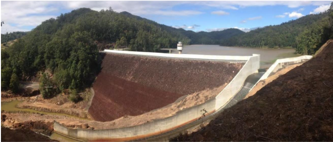
Figure 2-3 Panoramic view of spillway, dam wall and intake tower
