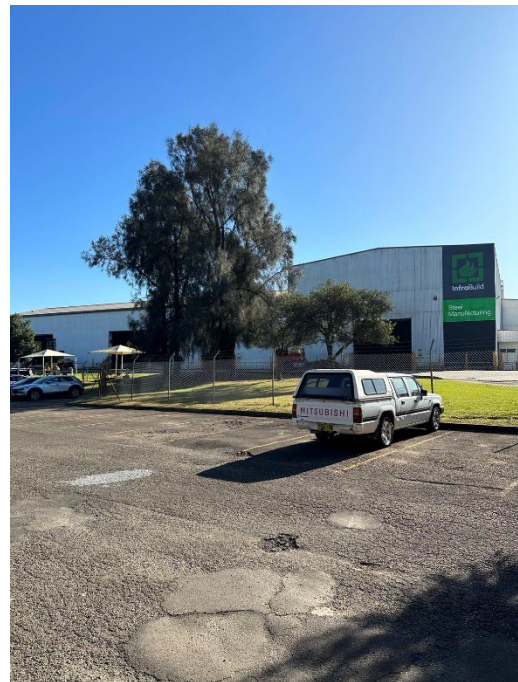
Picture 4 View of existing industrial building
