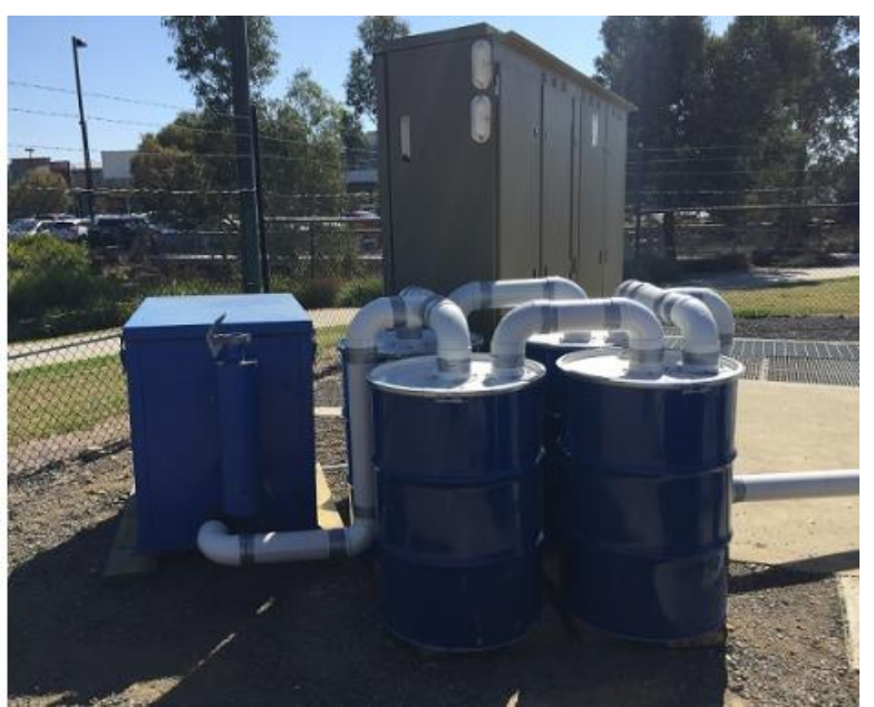
Figure 3.6 Granular Activated Carbon (GAC) Canisters for Air Filtration. Modular system allows all offensive gases to be scrubbed, and additional canisters on standby.
