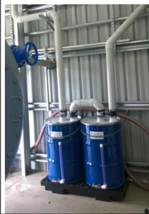
Figure 3.6 Granular Activated Carbon (GAC) Canisters for Air Filtration. Modular system allows all offensive gases to be scrubbed, and additional canisters on standby.
