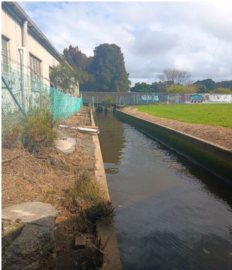
Below: North corner of the site along fence line: Concrete channel
