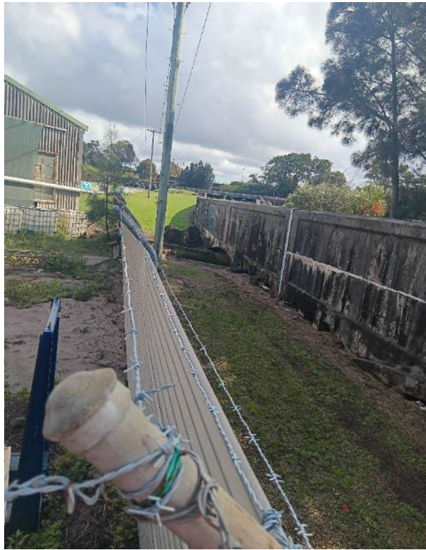
Above: North east side of site: Concrete Channel
