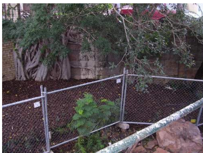
Photo 5: The purpose of the fence is to isolate the tree from the works and to protect the roots.
