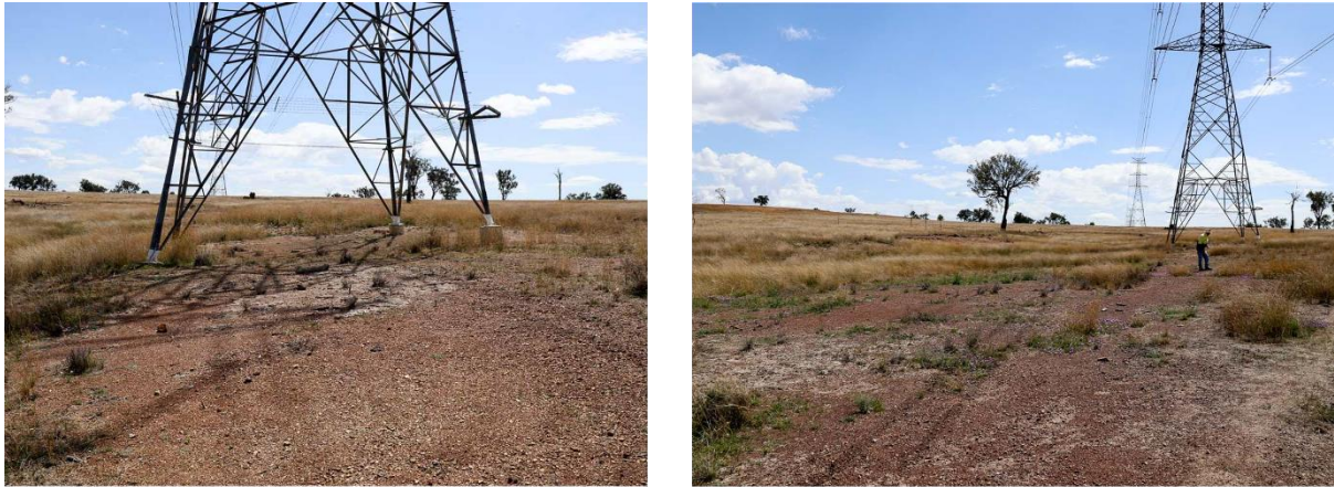
Erosion zones at base of Transgrid towers within easement
