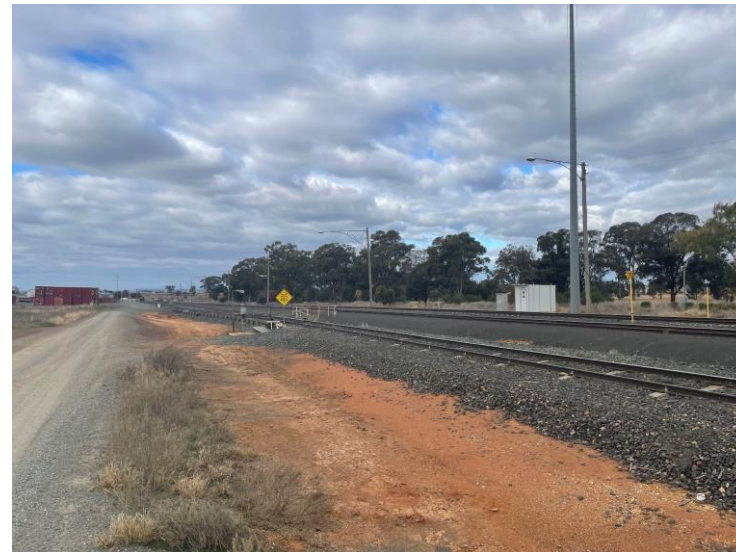
Figure 6.6 Goobang Junction looking east
