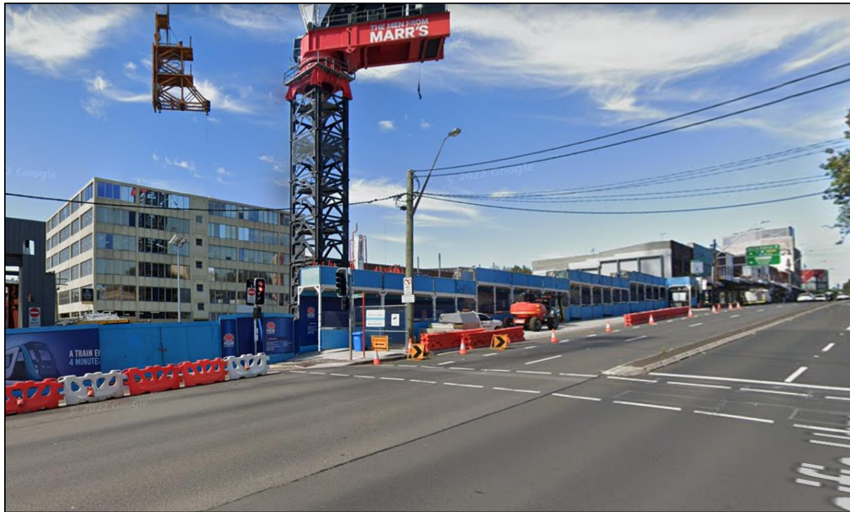
Figure 3. View South along Pacific Highway to Site B (Source: Google Street View, May 2023)
