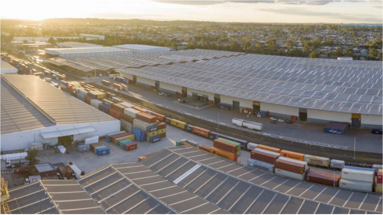
Picture 7 View over the intermodal facility looking north west.
