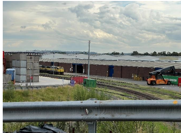
Picture 6 View from the overpass looking north west
