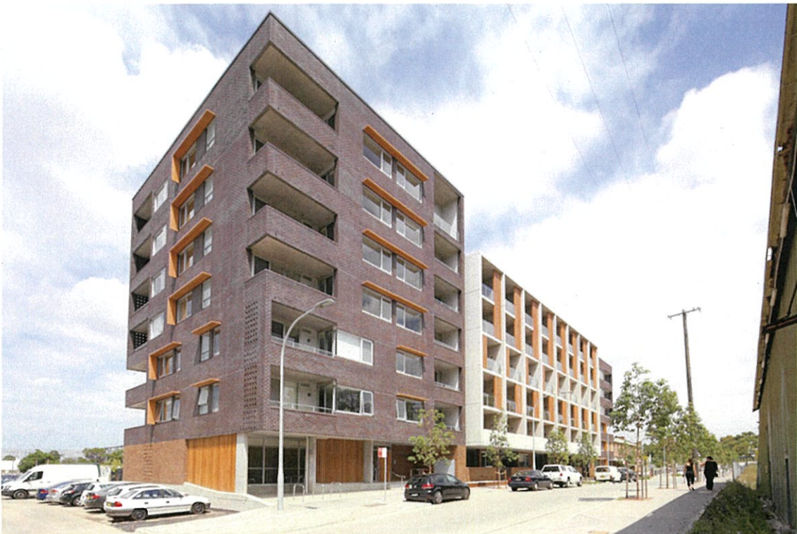
Figure 6 – Affordable housing development
