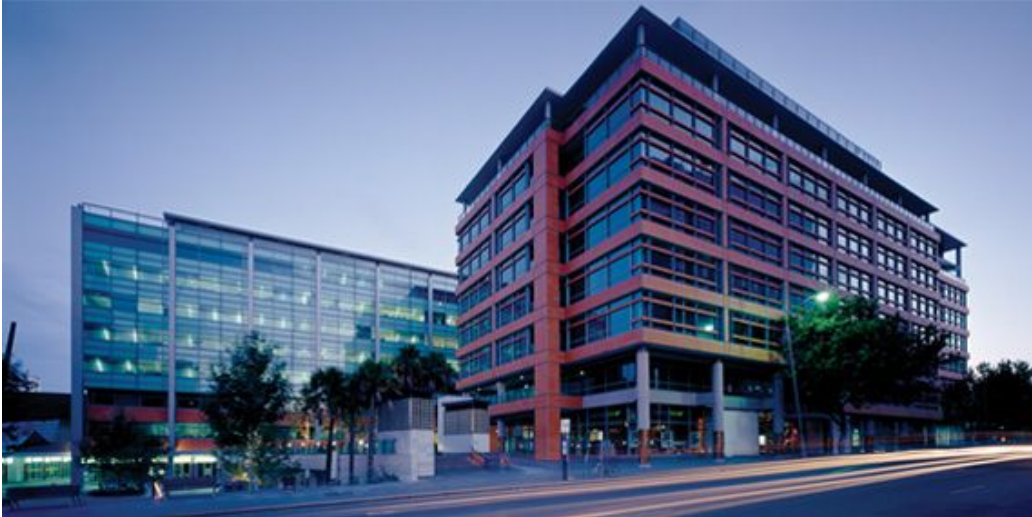
Figure 2 Henry Deane Plaza from Lee Street (14-18 Lee Street is the green glass building in the left, rear of the image)
