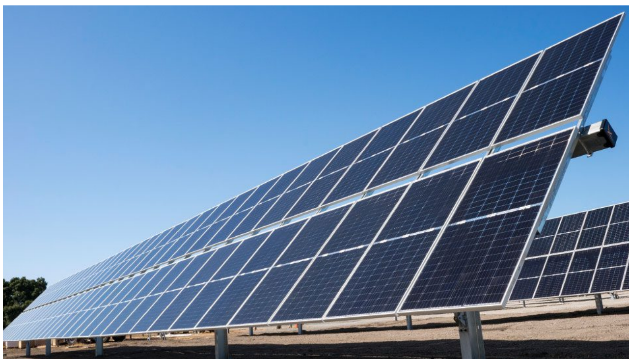
Plate 3.1 Example of a PV module layout (2 in portrait or 2P configuration)
