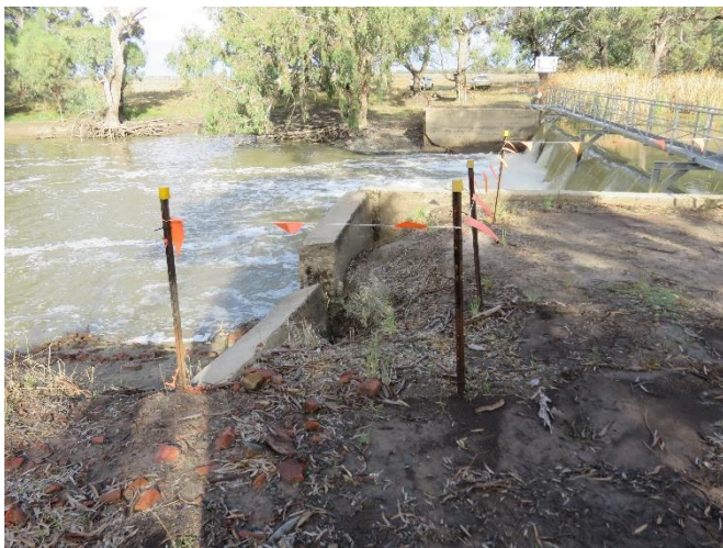
Figure 2-11 Examples of deterioration at the existing Hartwood Weir
