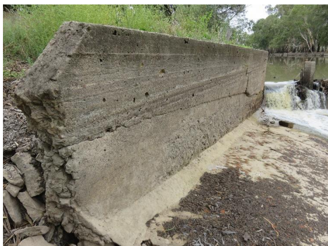
Figure 2-14 Examples of deterioration and missing drop boards at the existing Caroonboon Weir
