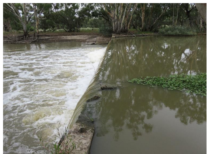
Figure 2-12 Examples of deterioration and missing drop boards at the existing Piccaninny Weir
