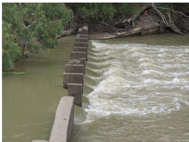
Figure 2-13 Examples of deterioration and missing drop boards at the existing Wanganella Weir
