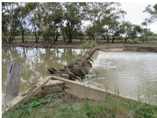
Figure 2-14 Examples of deterioration and missing drop boards at the existing Caroonboon Weir
