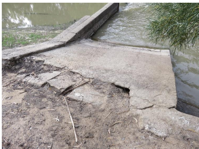
Figure 2-13 Examples of deterioration and missing drop boards at the existing Wanganella Weir
