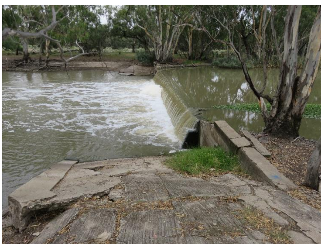
Figure 2-12 Examples of deterioration and missing drop boards at the existing Piccaninny Weir
