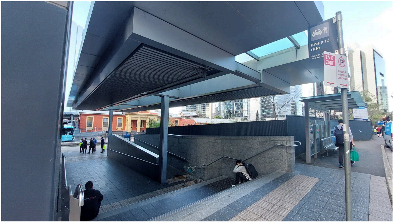
Figure 13 – View of the site’s through-site Footway connecting Argyle and Fitzpatrick Streets
