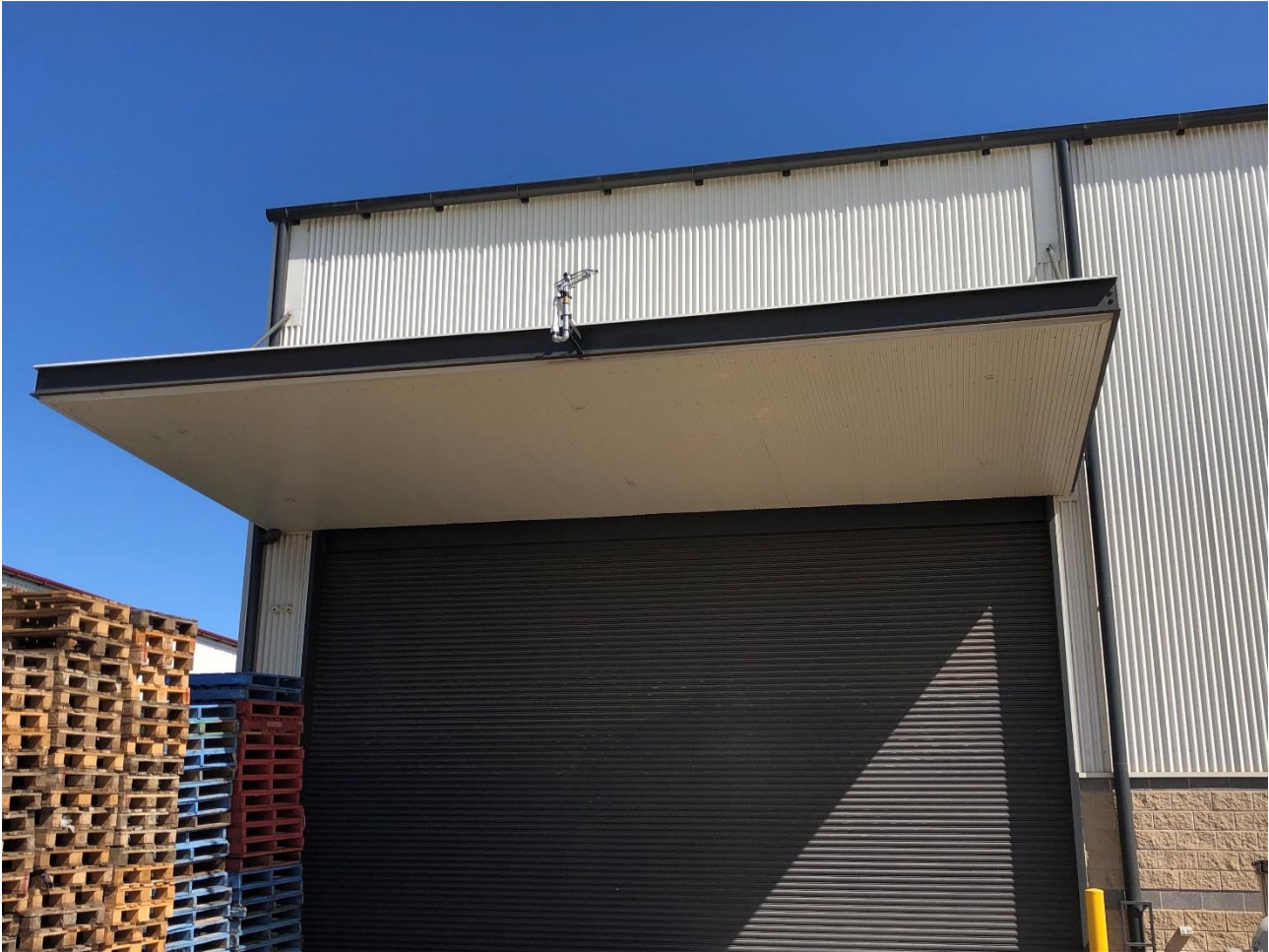
Photograph 2.3 Example of installed water cannon at southern boundary
