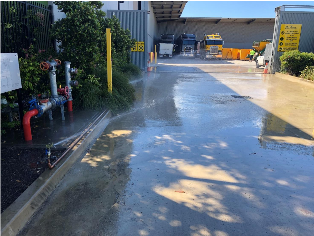
Photograph 2.2 Active wheel wash at site entrance
