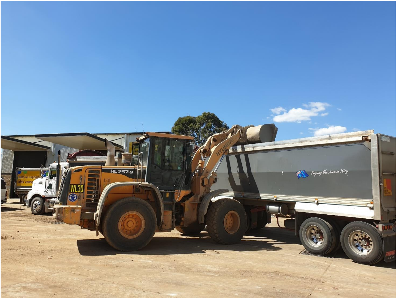
Photograph 2.7 FEL loading material to truck for export from site
