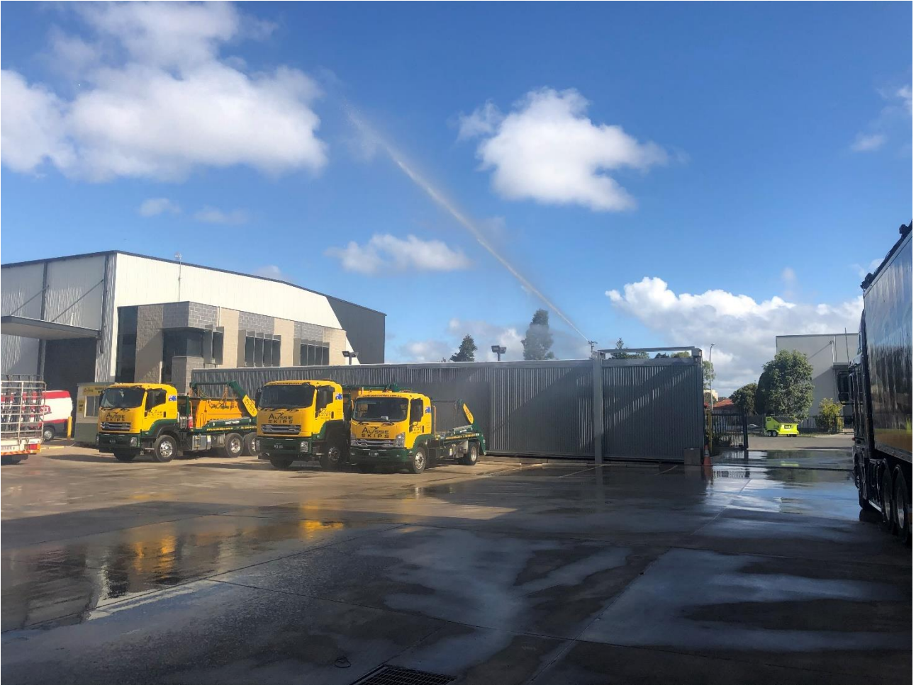
Photograph 2.4 Active water cannon at site entrance
