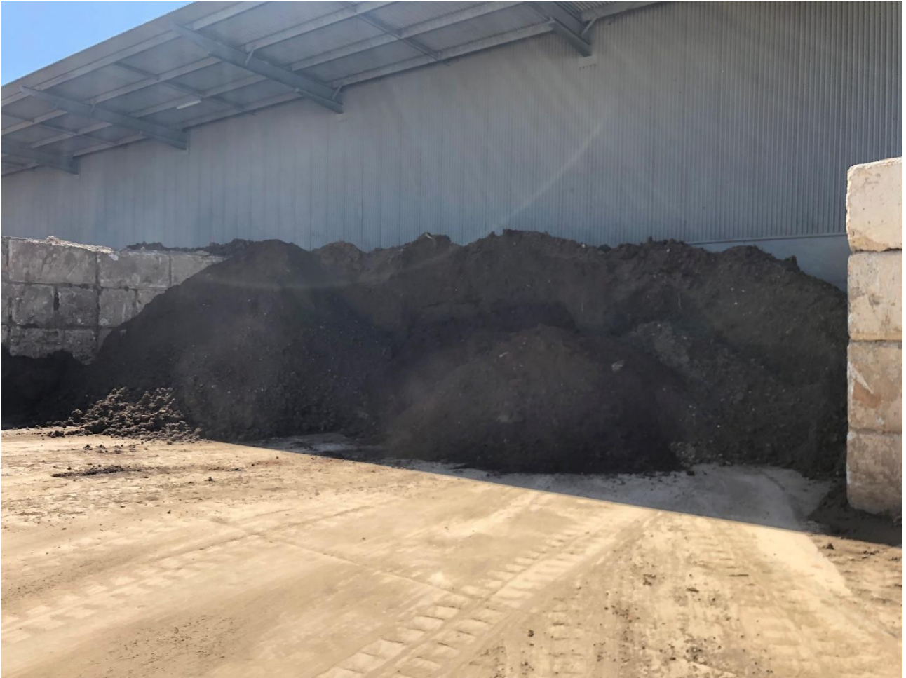
Photograph 2.5 Stored material in bunker at site (concrete block side walls and awning roof visible)
