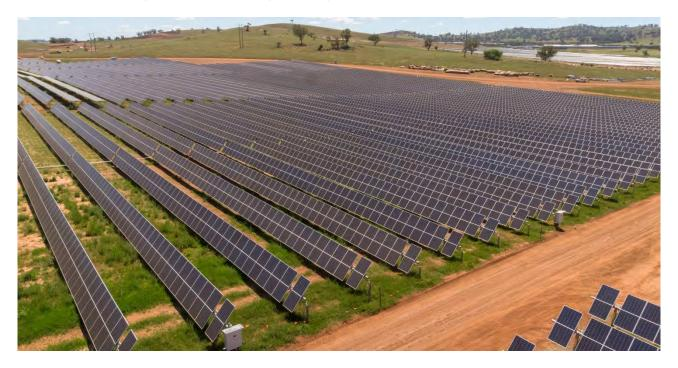
Plate 3.2 Example of a PV module layout – horizontal position
