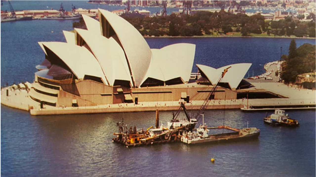
Figure 2-8 Construction of the Sydney Harbour Tunnel immersed tube tunnels in the early 1990s
