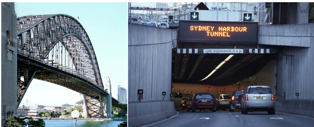
Figure 1-2 The Sydney Harbour Bridge (left) and Sydney Harbour Tunnel (right)
