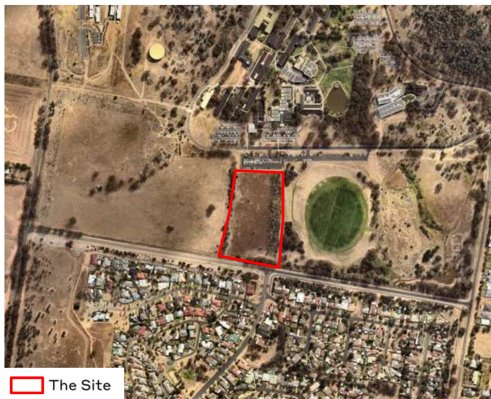
Figure 2 Aerial photograph of the site
