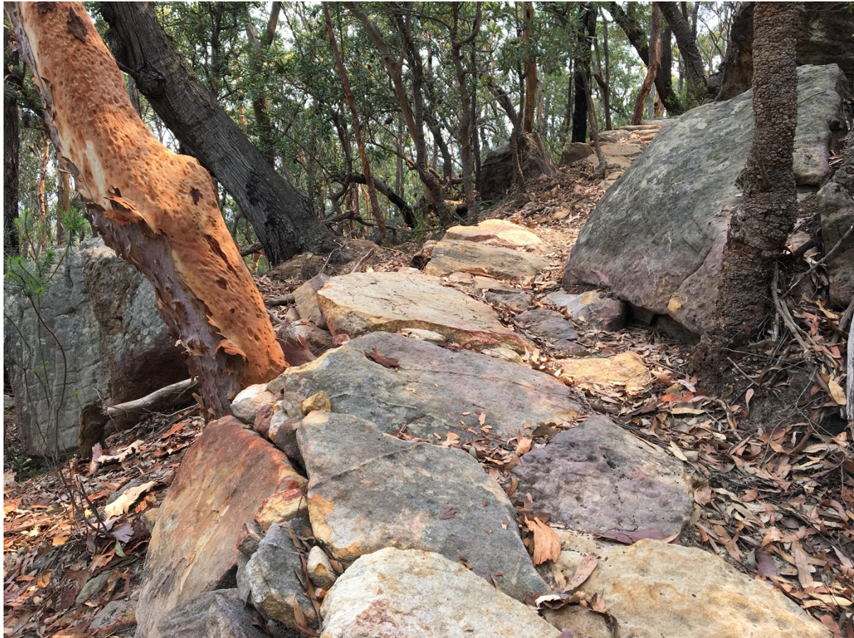
Figure 8 – Rock paving with onsite rock to protect an existing mature tree and affected rootzone (Location: Warimoo Downhill Track, Sydney NSW)
