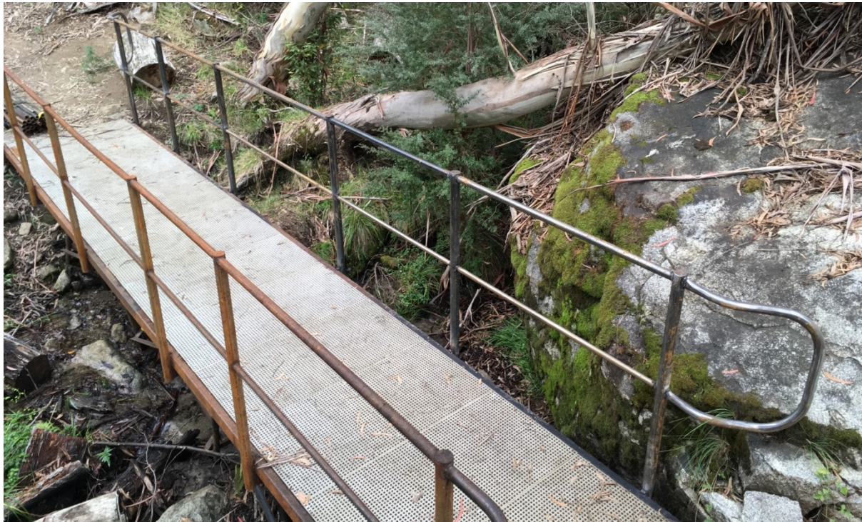
Figure 11 – Bridge structure with handrails to span over a deep and rocky gully (Location: Thredbo Valley Trail, Thredbo NSW)
