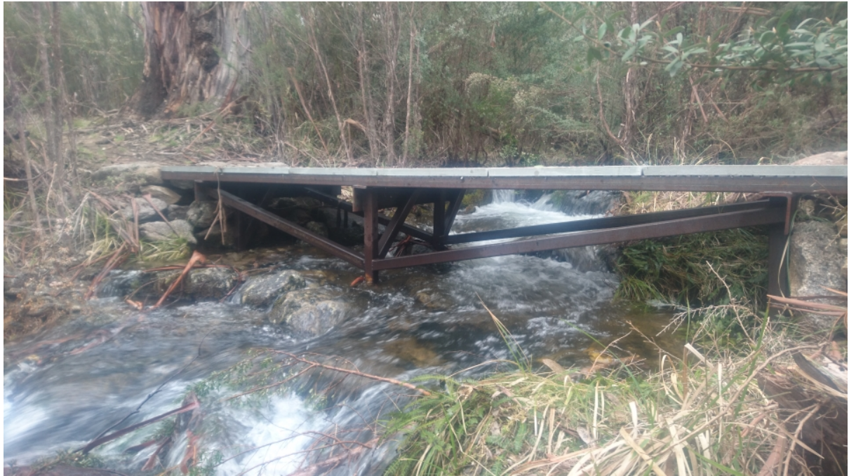
Figure 9 – Elevated FRP platform installed to cross an active watercourse (Location: Thredbo Valley Trail, Thredbo NSW)
