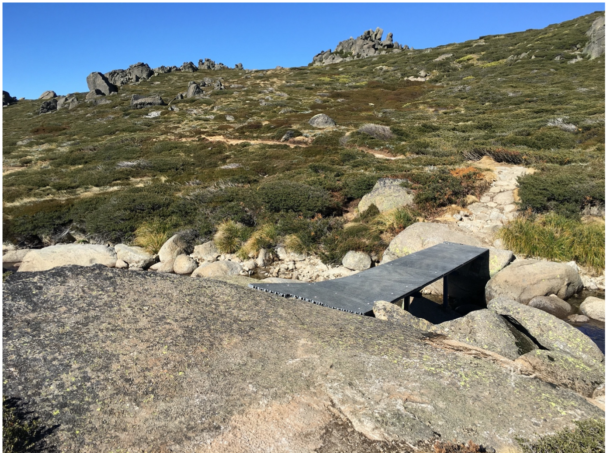
Figure 10 - Elevated FRP platform crossing between two rock slabs (Location: All Mountain Trail, Thredbo NSW)
