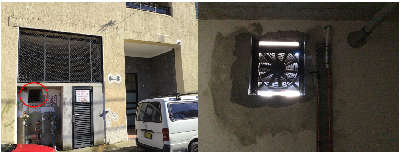
Figure 4. Ventilation grating on eastern wall
