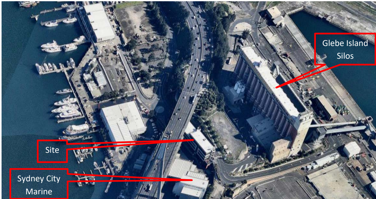
Figure 3: The Site and its locality looking west (Nearmap photo dated 02/07/16)
