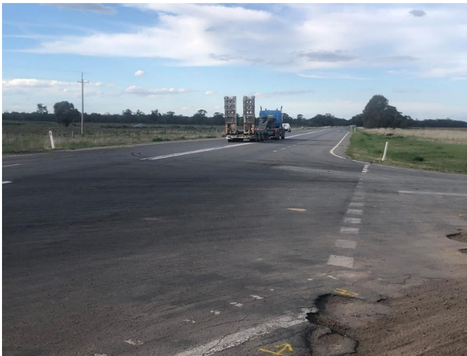
Figure 18 Donald Ross Drive intersection with Sturt Highway
