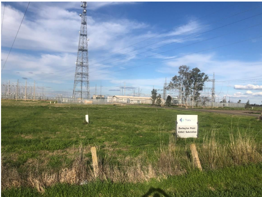
Figure 8 Darlington Point Substation
