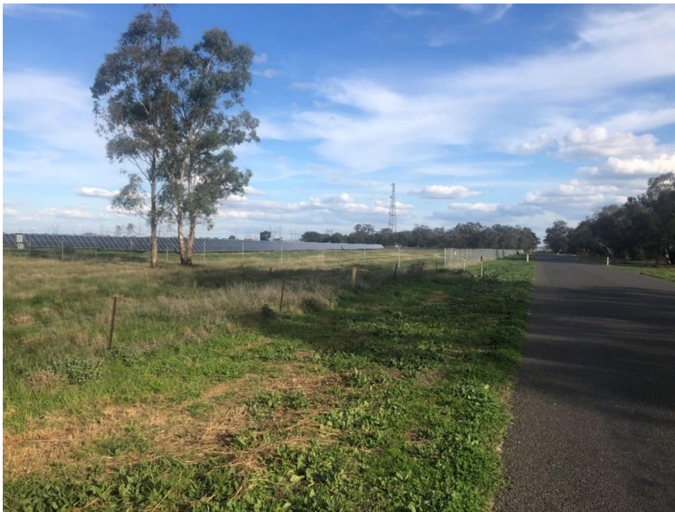
Figure 14 Darlington Point Solar Farm
