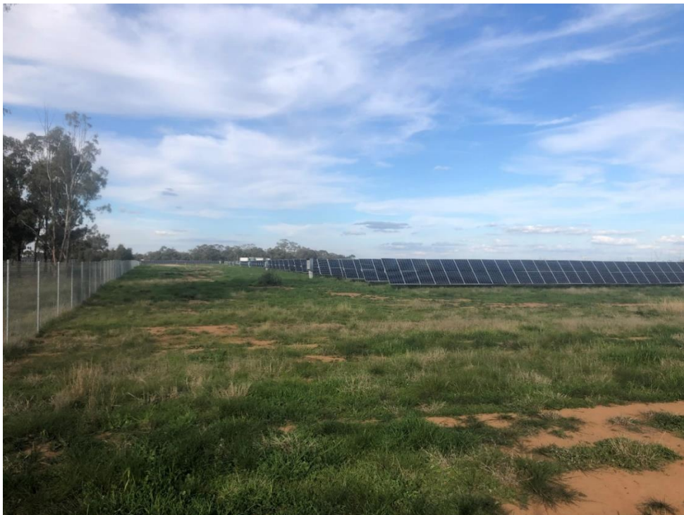
Figure 12 Darlington Point Solar Farm
