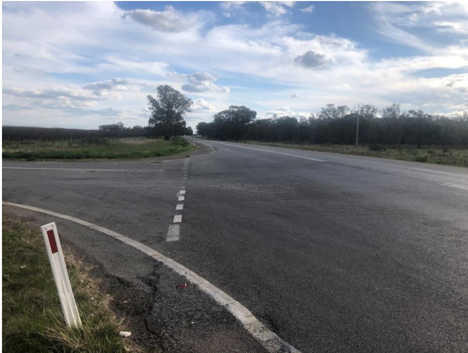
Figure 15 Donald Ross Drive intersection with Sturt Highway
