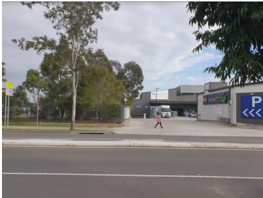
Figure 3 View of the school site adjacent to The Ponds Shopping Centre (facing west from The Ponds Boulevard) Source: Architectus (2021)
