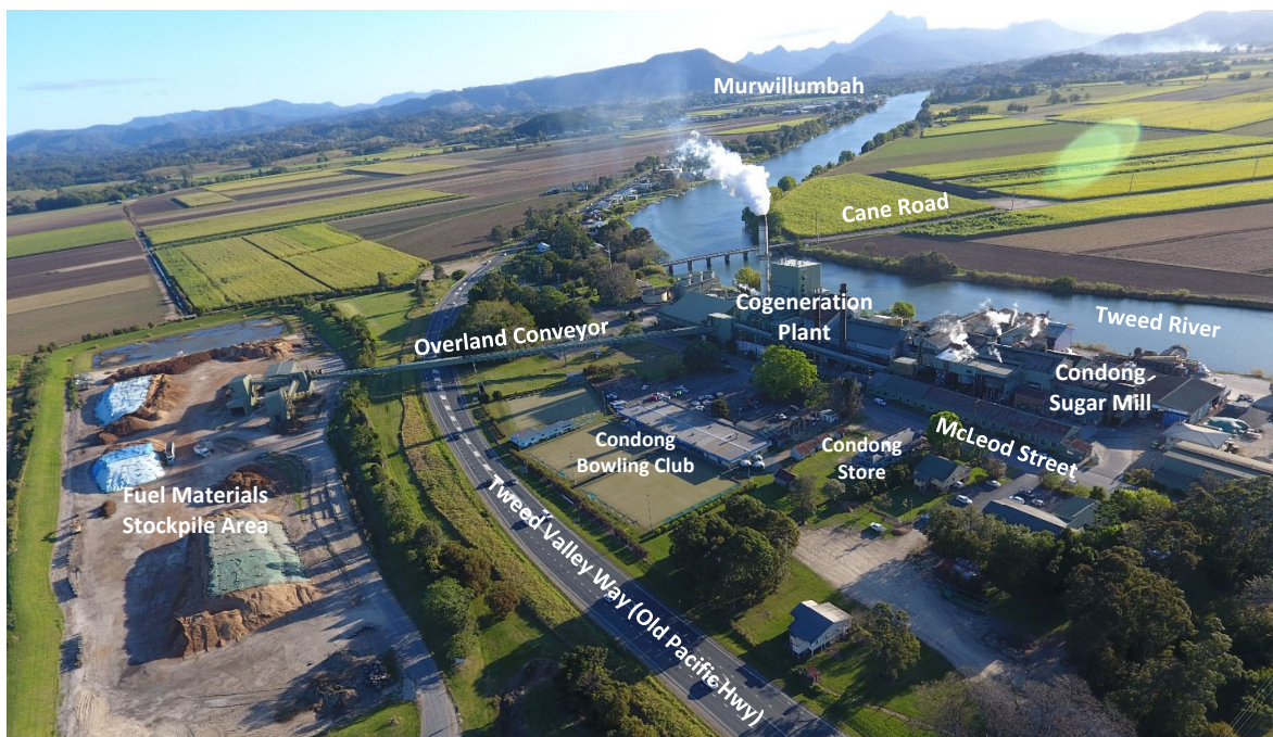
Photo 1 Condong Cogeneration Plant
