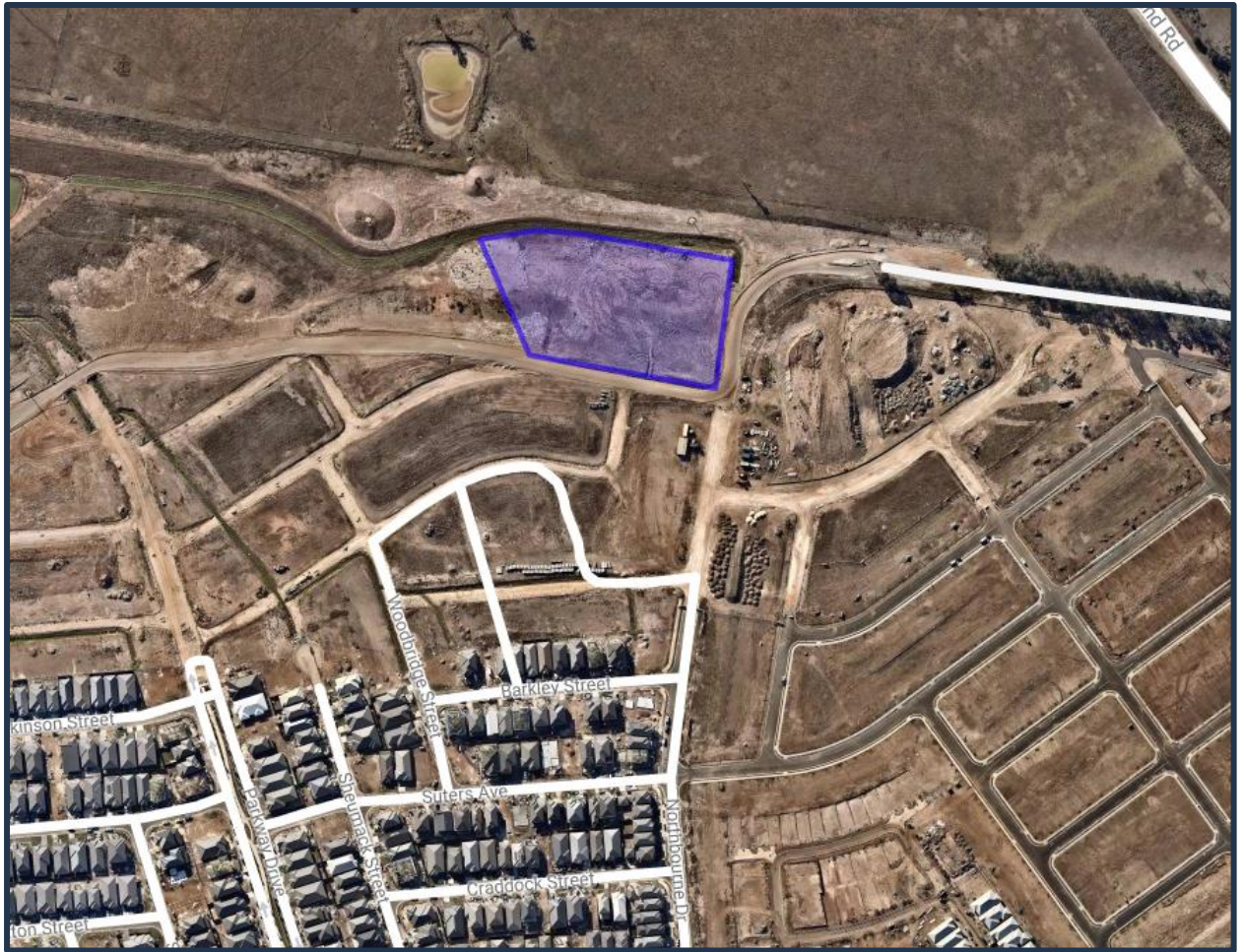
Figure 2: Site Aerial of Subject Site (Source: NearMap)
