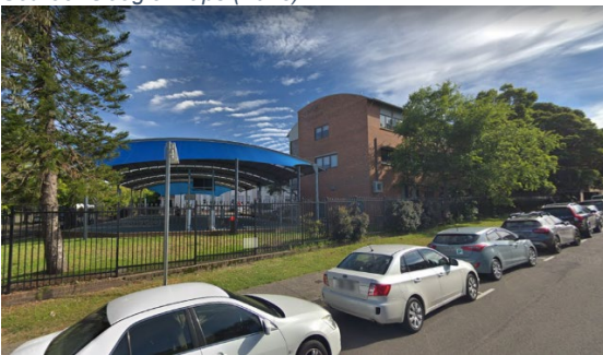
Figure 8 - Building A Heritage Listed Source: DJRD Architects Mosman Concept Design Report
