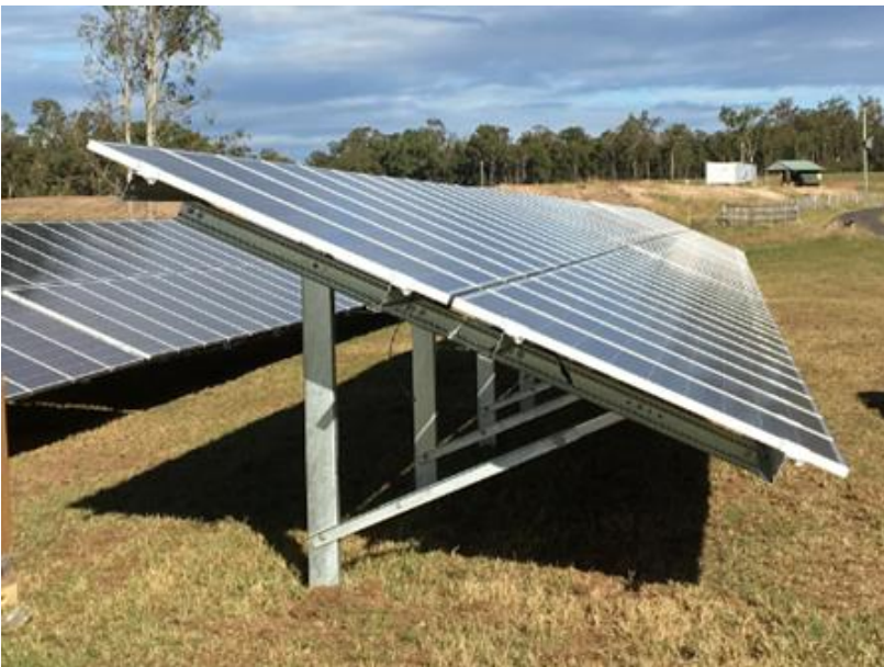
Figure 2-4: Example Ground Mounting Arrangements
