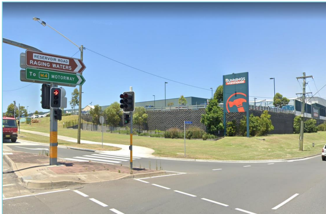
Figure 5 Bunnings Warehouse Blacktown – Reservoir Road
