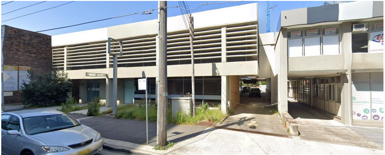
Figure 2 Site viewed from Restwell Street
