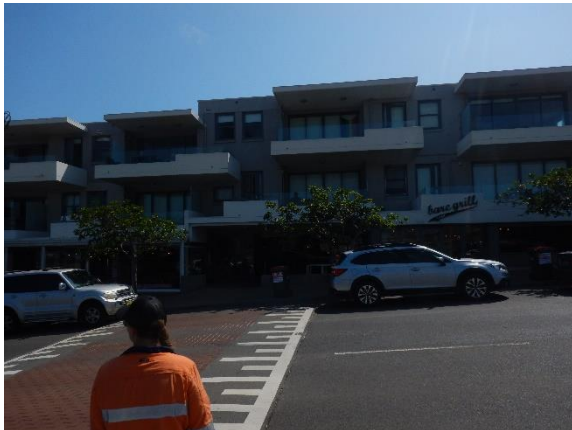
Figure 5.15: View north of buildings located in the northern portion of survey unit 3
