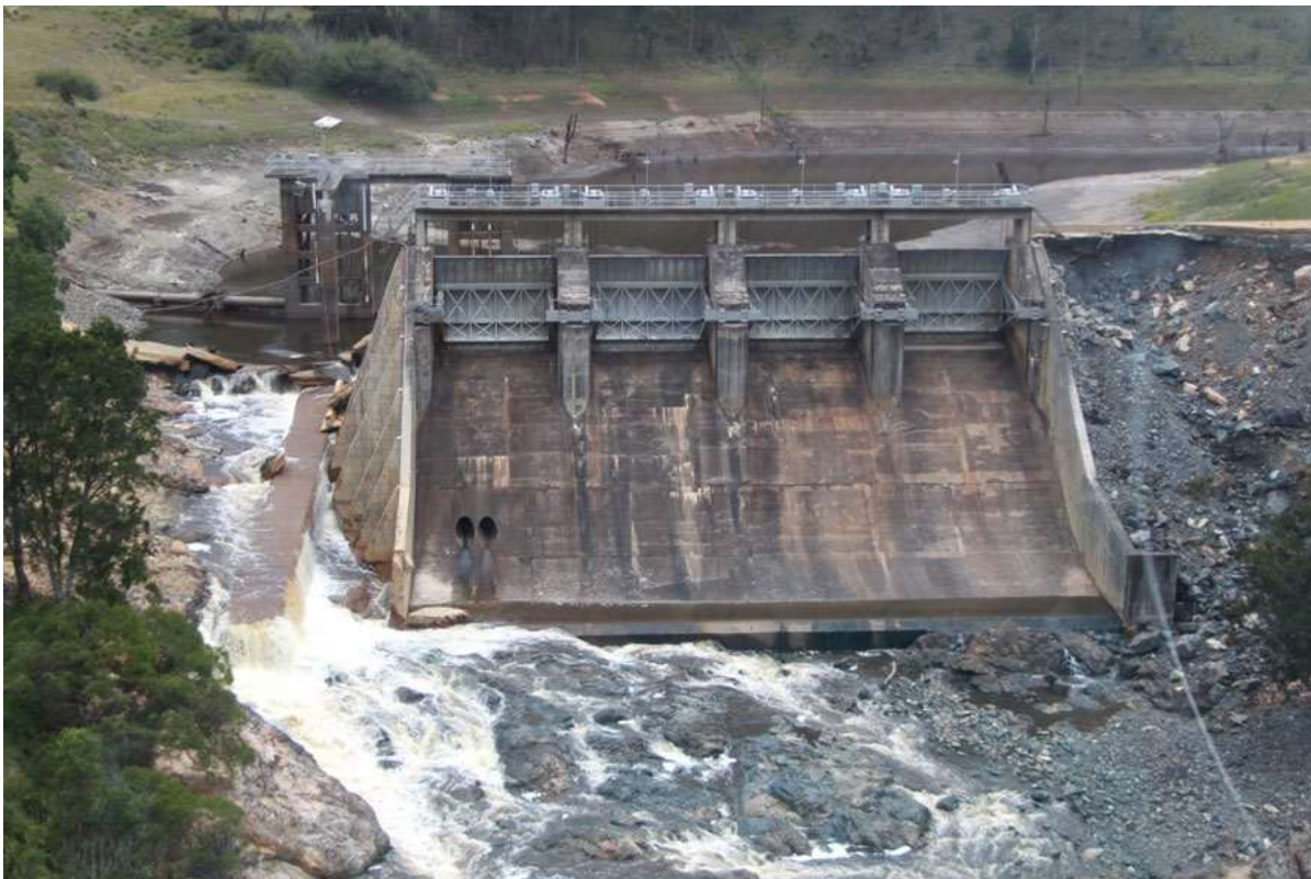
Figure 1-3 Oaky River Dam Post-Failure
